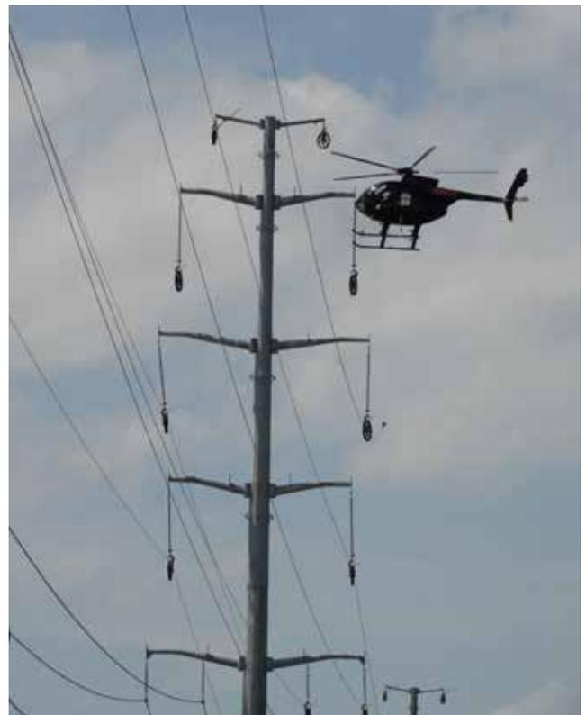
*A helicopter was used to string the lines between the poles. Aside from being more efficient and less invasive from an environmental standpoint, the helicopter work was fun to watch.*
